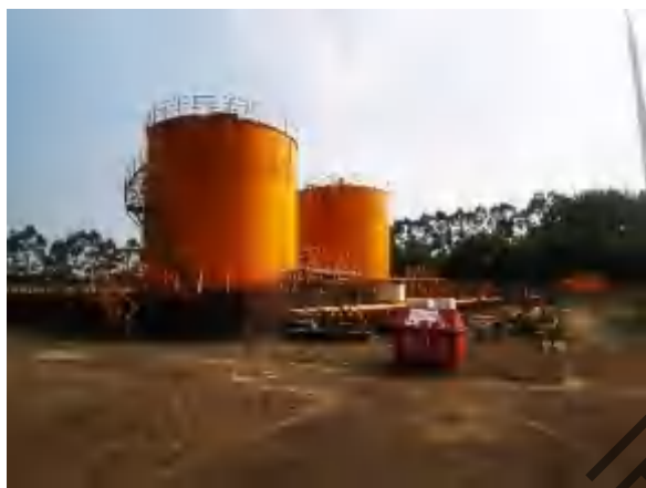
油罐、围堰、消防沙箱
